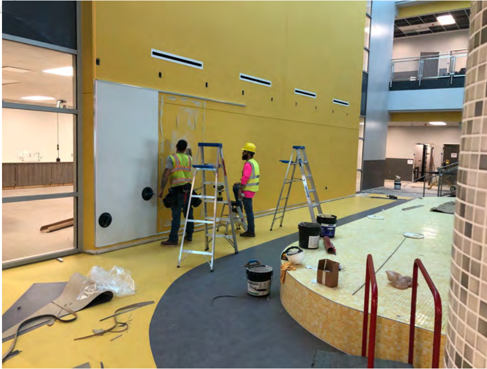
MARKER WALL INSTALLATION
